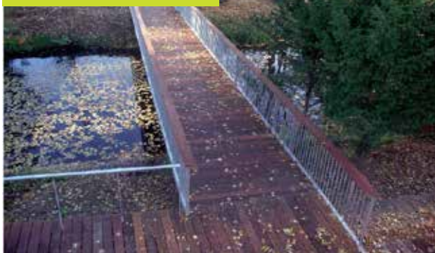
Balustres verticales, main courante bois
